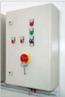
switch cabinet with control keys
