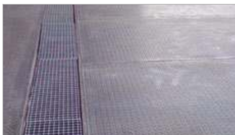
Gutter with grid
