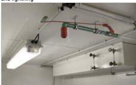
Emergency shower with 250 litre tank and explosion proof lightning
