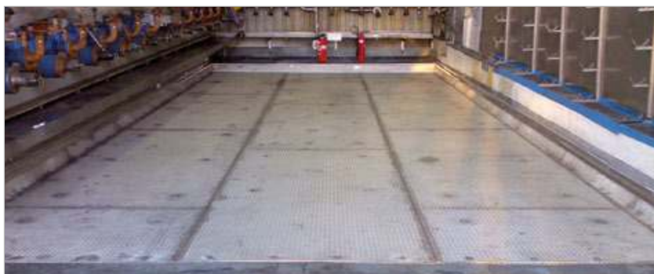
Ground protection lining made of stainless steel
