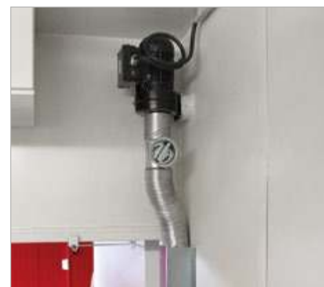
Explosion-proof ventilator
