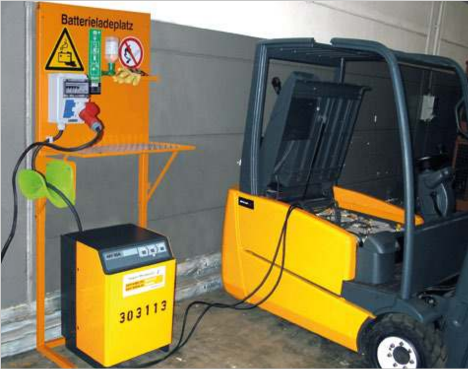
Type BL with fire extinguisher, with CEEform socket 400 V charging the battery of an electric forklift truck
